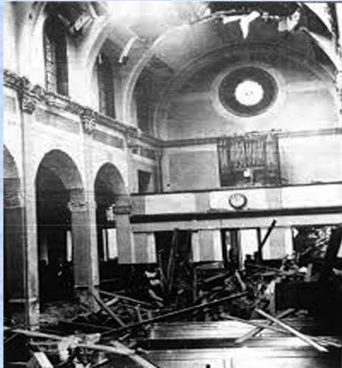
The bomb damaged St Peter' Church, Bradford, August 1940.
