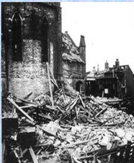
The bomb damaged St Vincent's Church, Sheffield, December 1940
